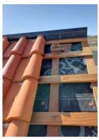
to check the underlayment while doing these repairs, because if the underlayment is deteriorated or will need replacement soon, then it may be advisable to replace the furring strips and underlayment at one single time in order to save on costs in the future.
