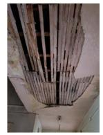
Sometimes where there are enough intermittent repaired cracks and/or missing sections of plaster, it will warrant a new plaster "skim coat" over the entire wall surface to give it a uniform texture.
