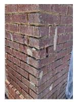
pointing operations. In some cases, other restoration of the building can be accomplished while a tuck pointing (due to expense) can be deferred to a short time after the initial restoration if it can be determined that water is not in fact infiltrating to the interior or into the masonry wall cavity.
