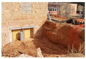
Sometimes replication of other lintels is desired to match original lintels, such as bricked arches, stone, precast concrete, or other types of lintels. For historic buildings, a newly installed window and/or door opening lintel will want to be differentiated from the historic lintels and the absence of a historic decorative lintel is one way to distinguish a new window and/or door opening.
