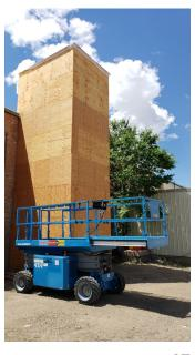
elevators, the pit depth is generally approximately 5 feet deeper than the existing lowest floor level of service, which can cause shoring and undermining of existing foundation concerns as well as waterproofing concerns; all of which can be expensive to mitigate. Sometimes, concrete admixtures can be added to the concrete foundation of the elevator pit to mitigate the waterproofing concerns.
