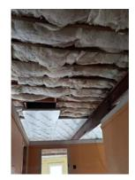
in the walls. Adding insulation on the upper side of the roof can be beneficial when an exposed structure is desired on the interior.
