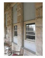
which can give the appearnace of glass on the exterior and a wall can be installed on the interior to block the window from the interior side, but note to properly insulate the cavity between the window and the wall in this scenario.
